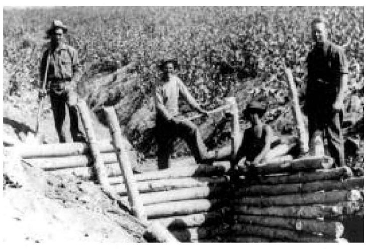
CCC workers in Hobbie Creek Canyon east of Springville worked to build a log dam for soil conservation.
